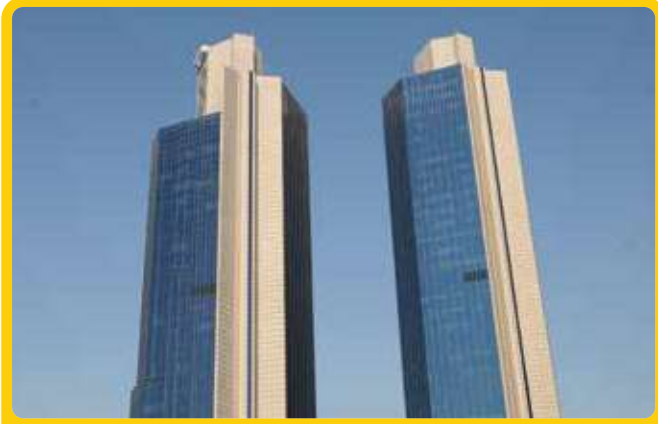
Sabancı Center – İstanbul, 1991
